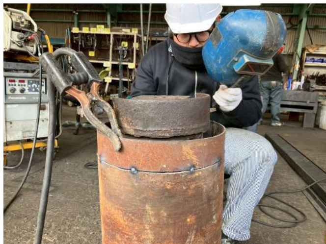
損傷箇所溶接補修②
